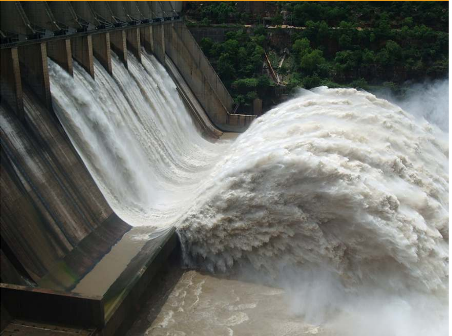
Figure 20.1 Electric energy in massive quantities is transmitted from this hydroelectric facility, the Srisaïlam power station located along the Krishna River in India, by the movement of charge—that is, by electric current. (credit: Chinto here, Wikimedia Commons)
