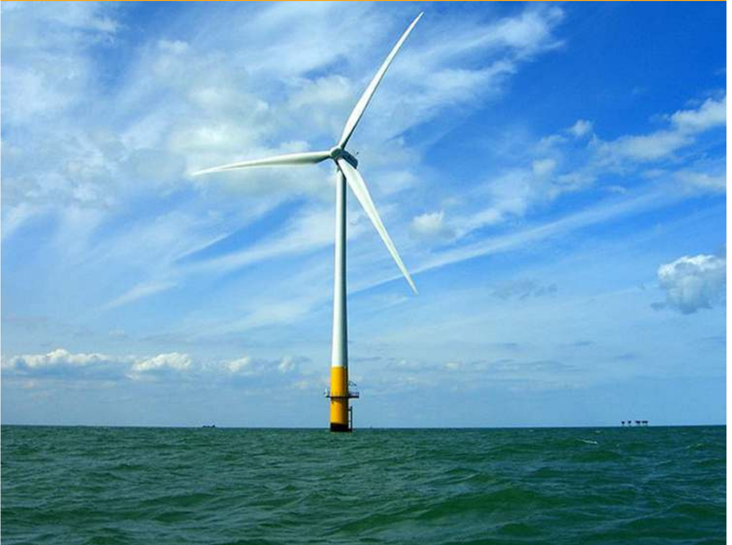
Figure 23.1 This wind turbine in the Thames Estuary in the UK is an example of induction at work. Wind pushes the blades of the turbine, spinning a shaft attached to magnets. The magnets spin around a conductive coil, inducing an electric current in the coil, and eventually feeding the electrical grid. (credit: phault, Flickr)
